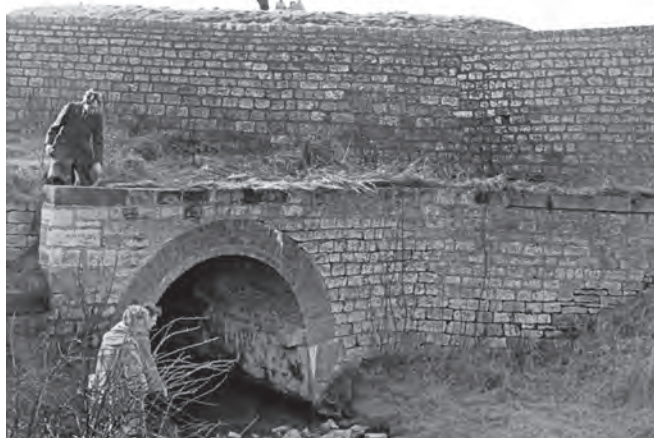
The eastern portal of Norwood Tunnel in 1959.
